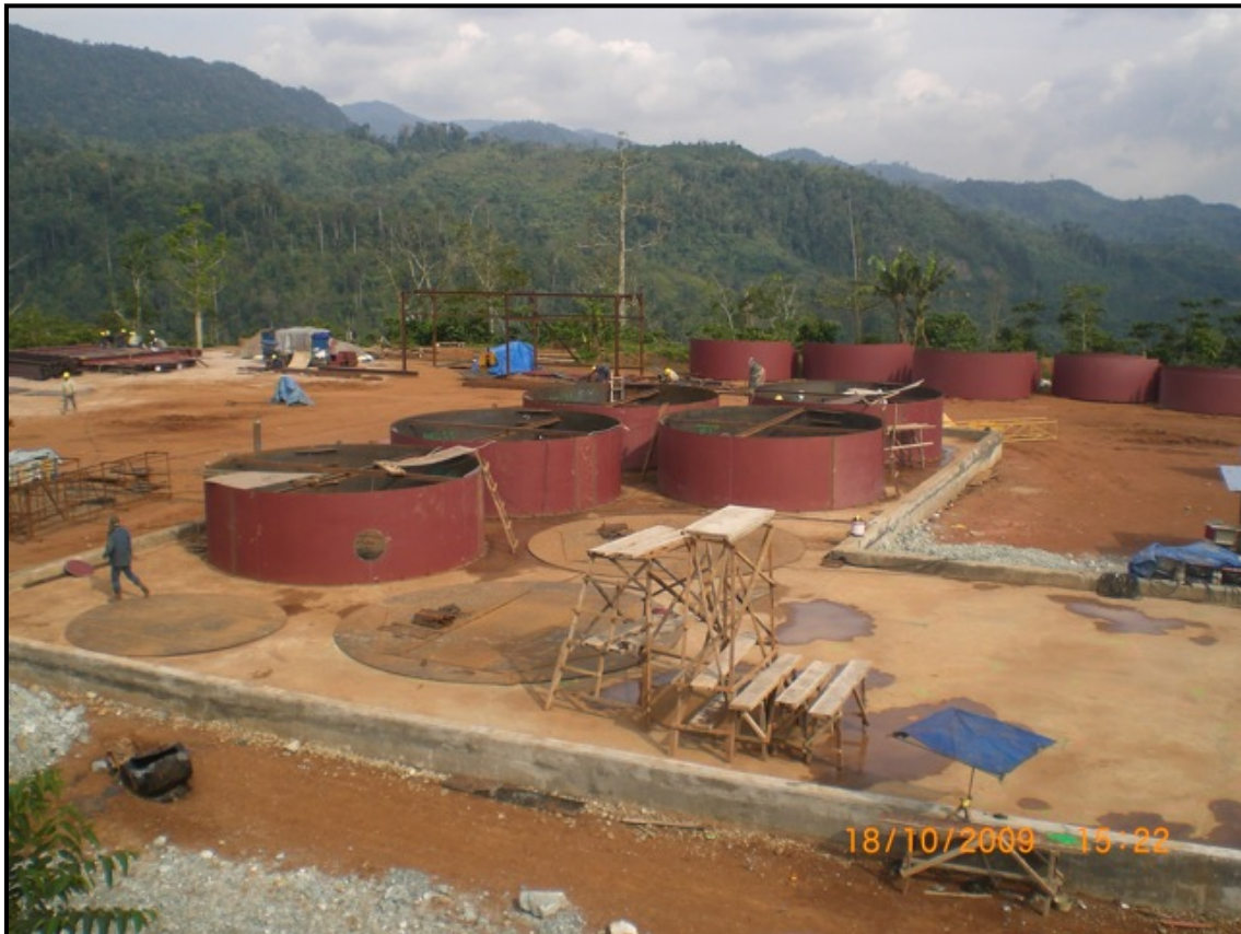
Plate 2. Way Linggo process plant leach tanks under construction
