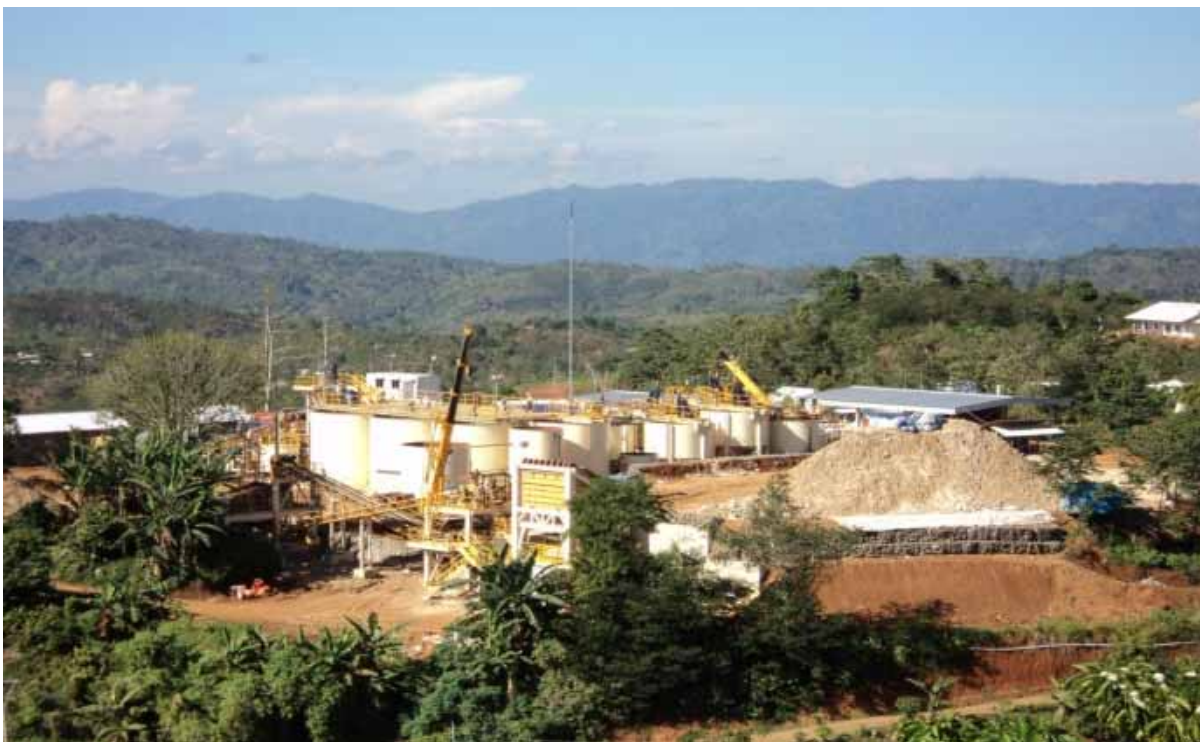
Figure 2 – Way Linggo 400 tonnes per day Merrill Crowe gold plant.
