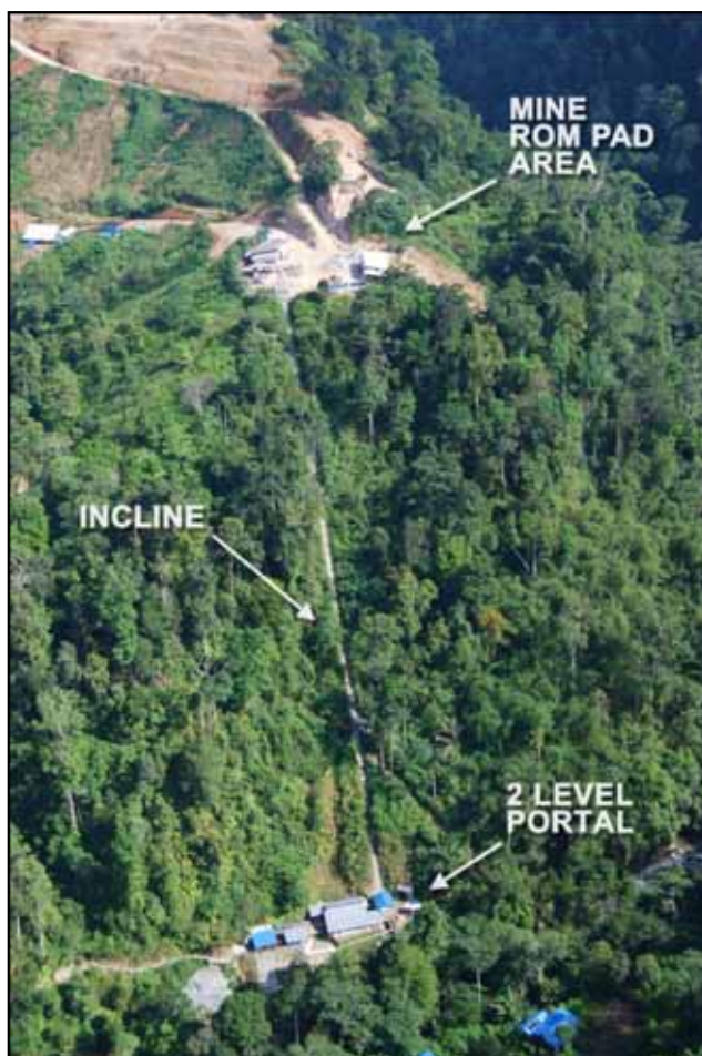
Figure 5 – Aerial view of Way Linggo minesite showing mine service area, level 2 Portal and incline.
