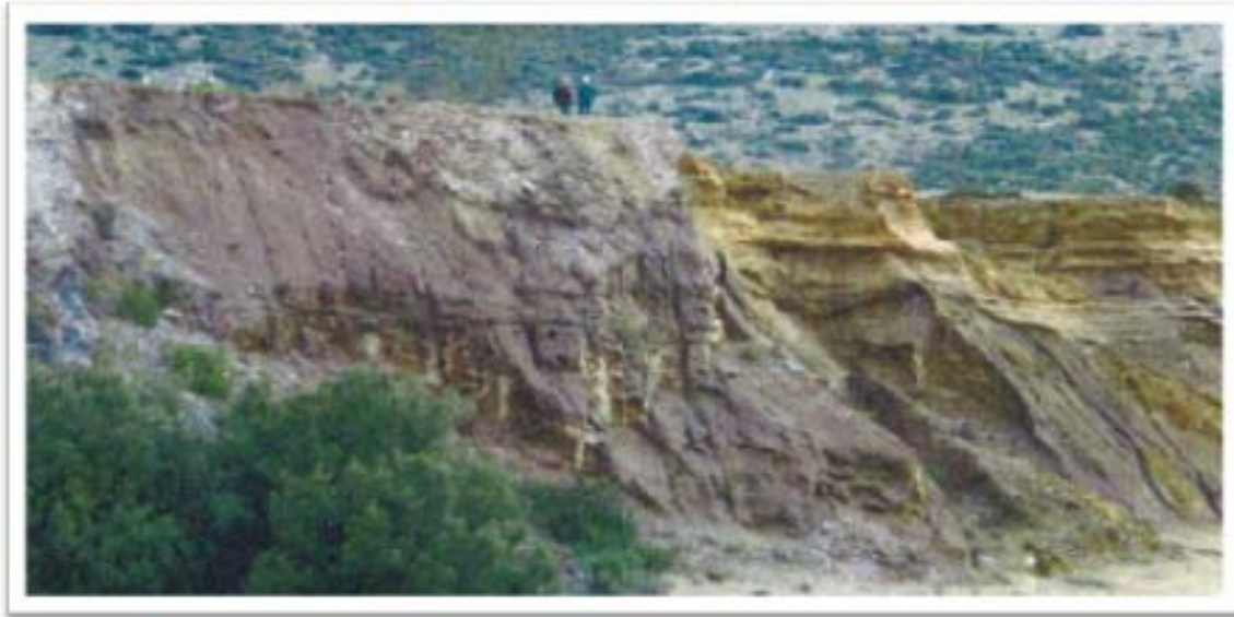
Picture showing an eroding tailings dam (Dam 2) located in Montevecchio.
