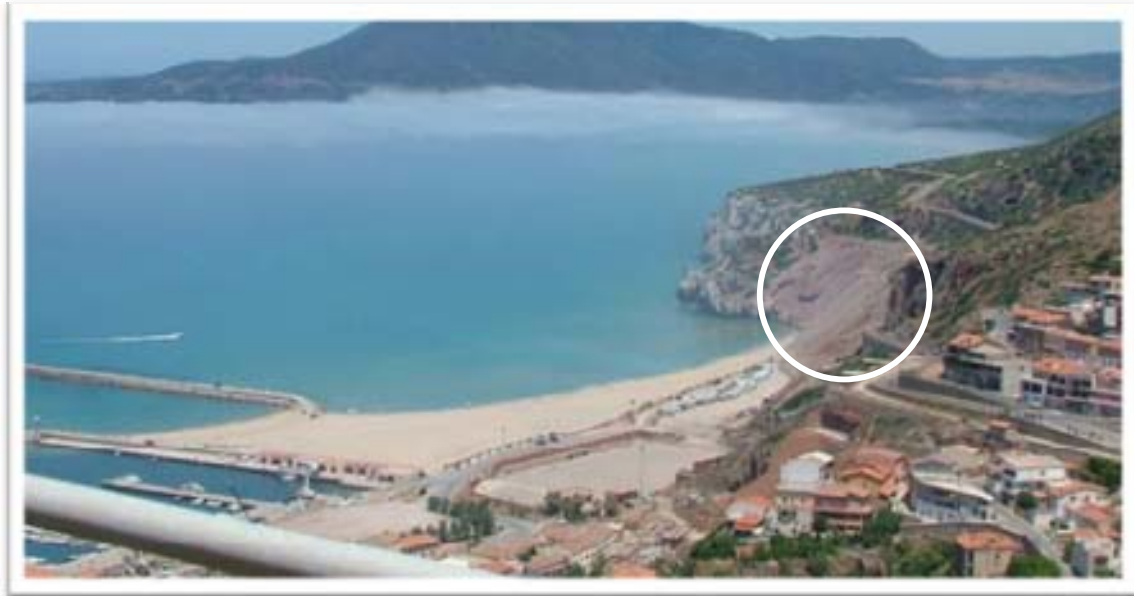
Picture showing Buggerru Marina – tailings are located in the Marina (bottom left of picture) and on side wall (circled).
